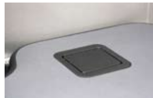
Pop-up units include Ethernet network and parallel ports as well as standard AC power outlets and can be customized to a site's particular needs.
